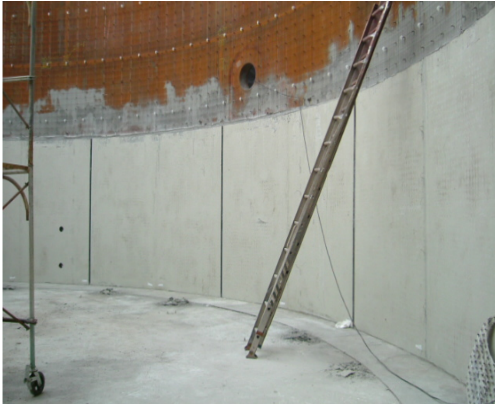
1st Section Back-filled with Concrete After The Removal Of The Shuttering
