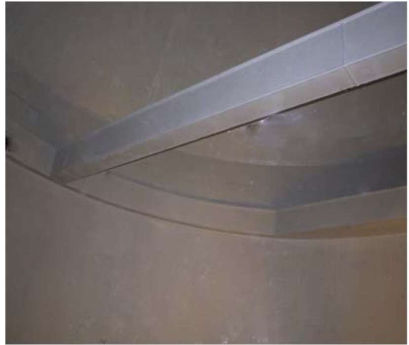
Finished Polypropylene Lining
