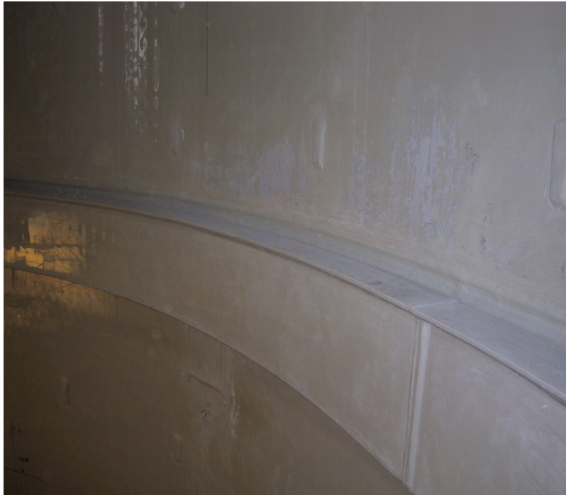
Finished Polypropylene Lining
