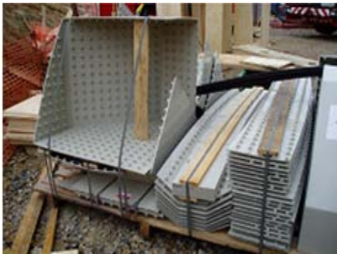
Lining for the support ledge
