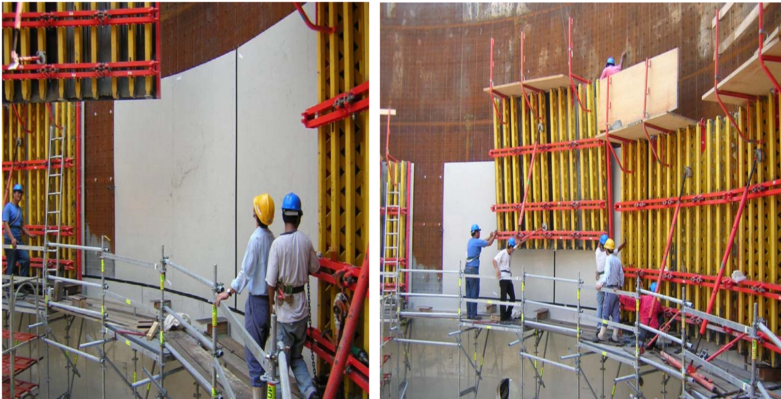
Placing of 2 nd Section
