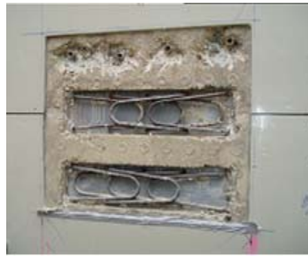
Reinforced Tie-ins designed to swing 90 degrees from structure wall
