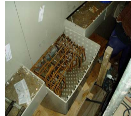
Additional rebar welded onto tie-ins for structural support
